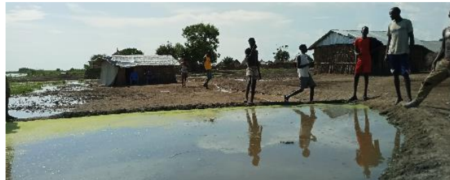
Dyke construction to prevent water from flooding the school
