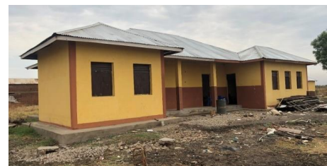
Nasir County Education office rehabilitation
