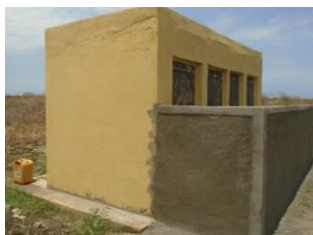
Toilet block in Nasir
