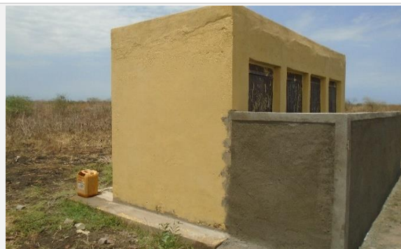
Toilet block in Nasir
